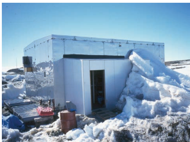
Photo 8 Gravimeter room at Syowa Station
