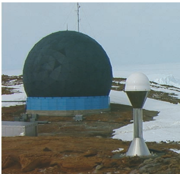
Photo 12 Multipurpose antenna at Syowa Station (In the redome at the back, the GPS continuous observation station is at the forefront.)
