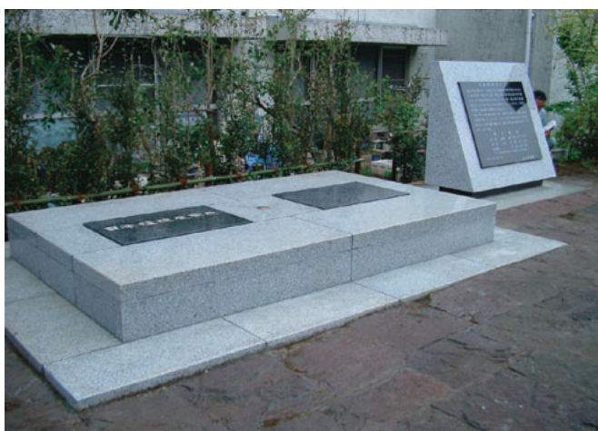
Full view of Horizontal Origin Point of JGD2000 and its metal marker in Tokyo
